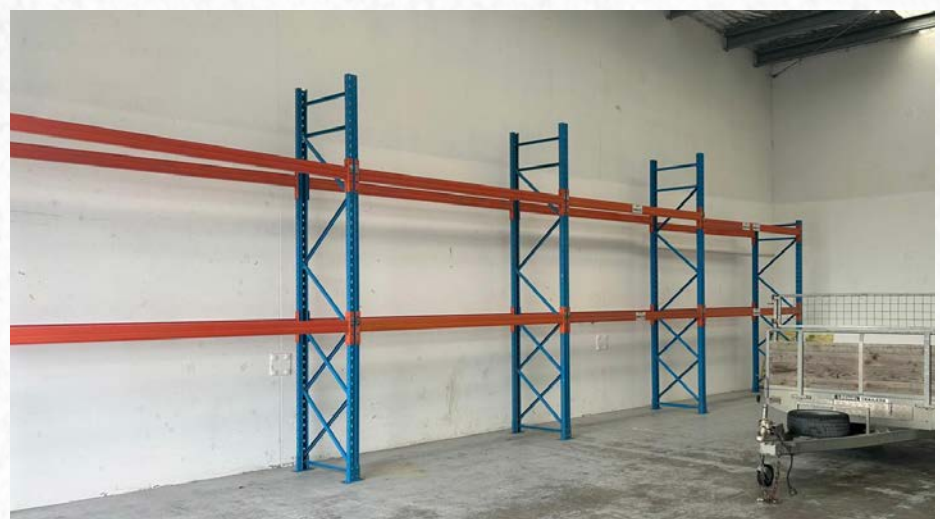
Pallet racking being set up in Greymouth.
